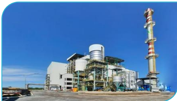
Vietnam Hau Giang WTE Project Supply, installation and testing of an incineration grate furnace and a leachate treatment system
